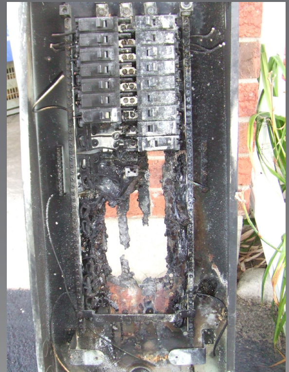
120/208 volt 3 phase panel. Cause not known, however history of hot spots. Causes downtime for general power.
