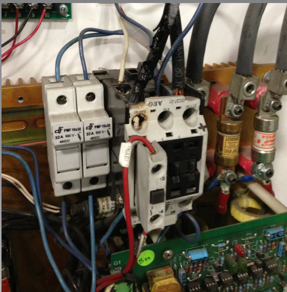
Motor contactor, causes downtime for a production line.
