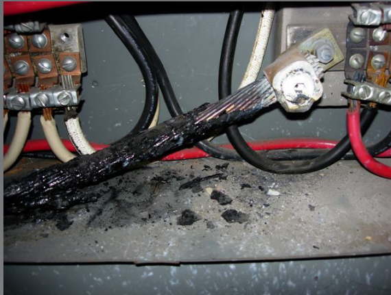
600 volt splitter, causes downtime for general power
