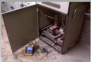
Power Quality Analyzer, enables us to monitor how well your power is doing. Power quality is a measure of how well a system supports reliable operations of its loads.
